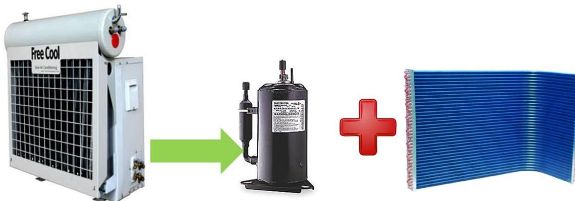
1- Stage Compressor and condenser coil.
